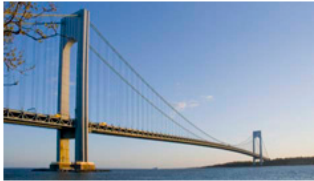
Denys's Ferry was located near the Brooklyn end of the Verrazano Narrows Bridge (Rick Shwab)
